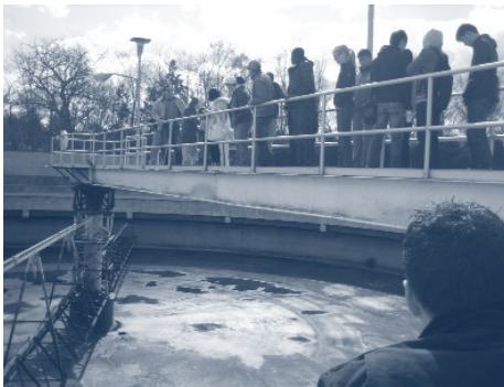
Standing on the walkway over the final clarifiers
